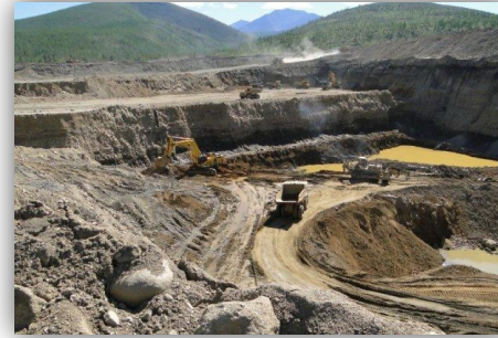
Shubarkol Komir Coal Processing Plant Kazakhstan, 2018
